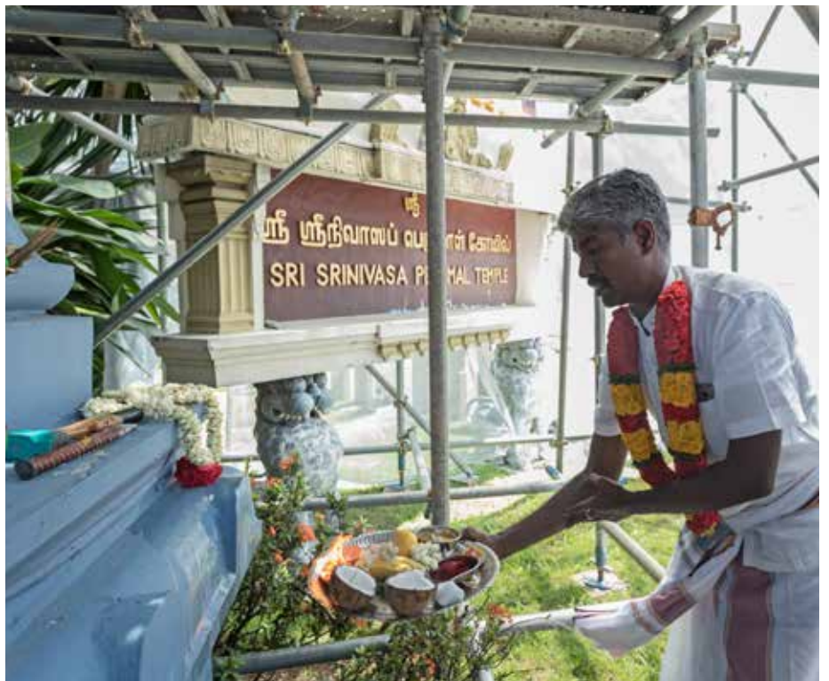
Chief Sthapathy, Mr S Anand, performed a ceremonial prayer to start the redevelopment works for the Rajagopuram and Vimanams.
